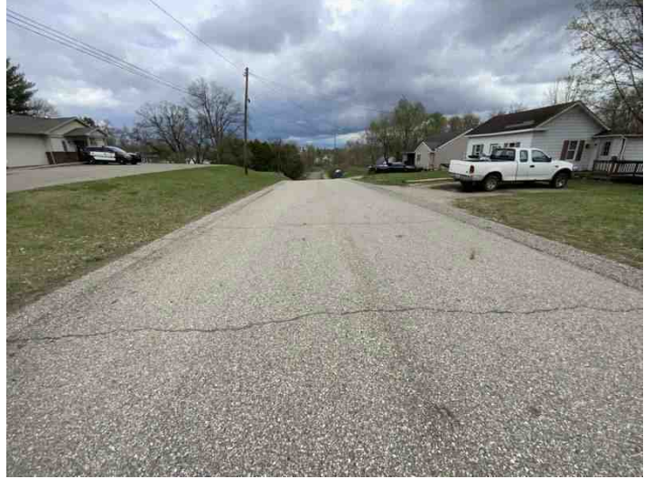
Lake Street Looking East
